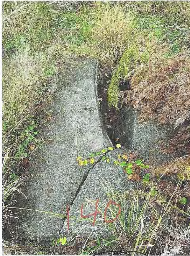
Pond 140 Outfall – Repair cracked structure. Clear Vegetation
