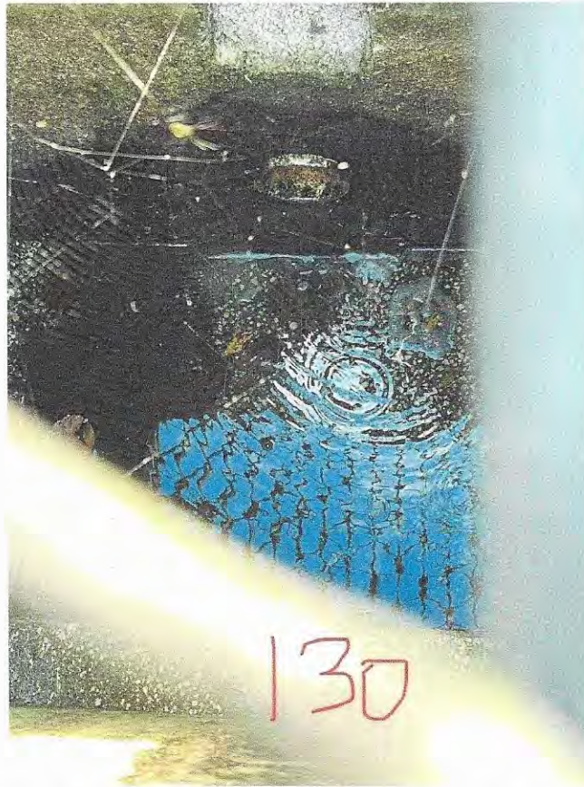
Pond 130 Control Structures - Repair crack in structure wall. Water observed leaking through outfall structure wall.
