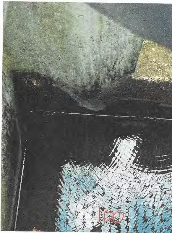
Pond 100 Control Structures - Re-grout where the Bleed-Down pipe was plugged. Water observed leaking through outfall structure wall.
